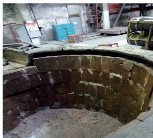
Figure 2. Lining of the ladle for casting ferrochrome grades FeCr 600–650.
